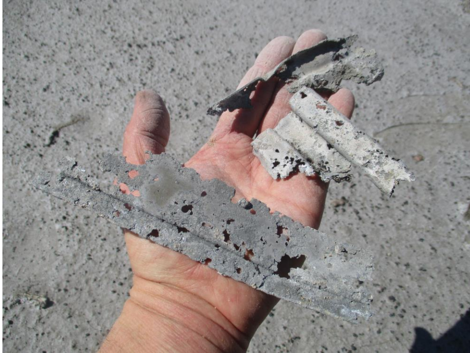
More parts full of holes from corrosion
